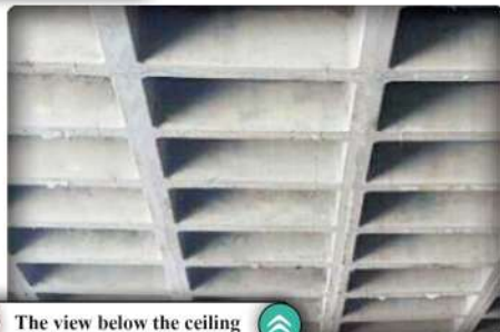
The view below the ceiling
