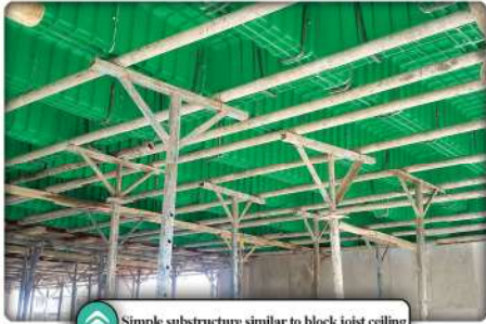
Simple substructure similar to block joist ceiling
